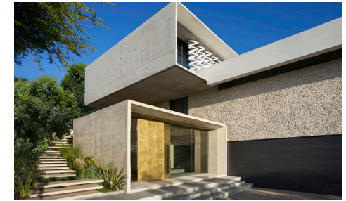
off-shutter concrete wall
