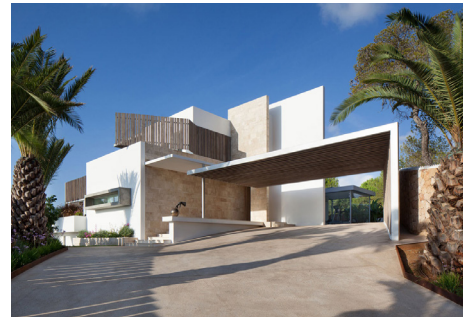
carport attached to main dwelling
