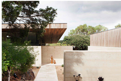
rammed earth walls
