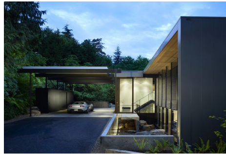
carport attached to main dwelling
