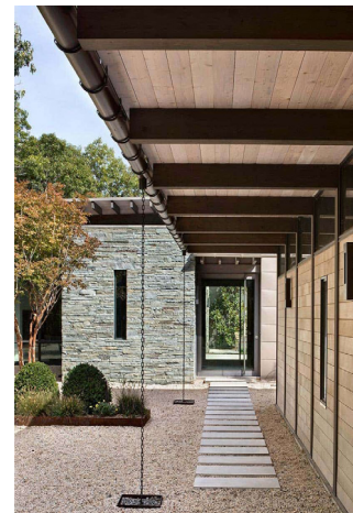
exposed half round gutter
