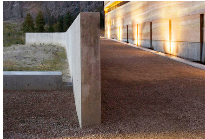
rammed earth walls
