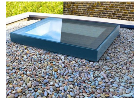
skylights within roof plane
