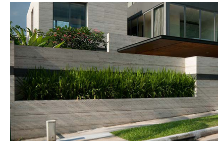
travertine stone boundary wall
