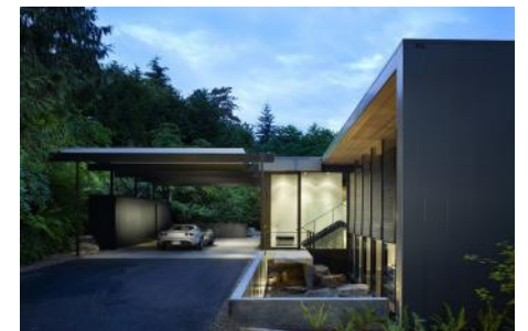
carport attached to main dwelling
