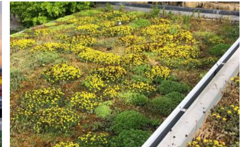
extensive green flat roof
