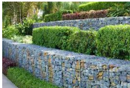
Gabion retaining wall
