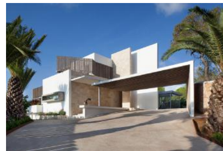
carport attached to main dwelling
