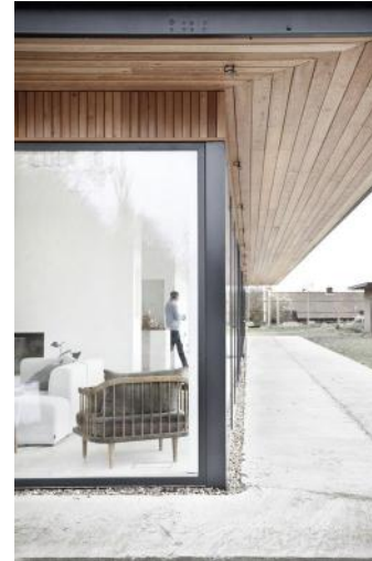
slatted timber eaves
