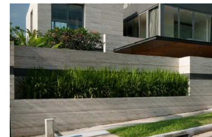
travertine stone boundary wall
