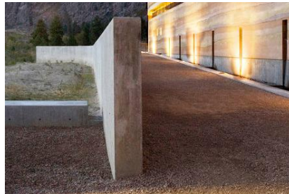
rammed earth walls
