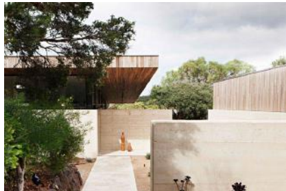
rammed earth walls
